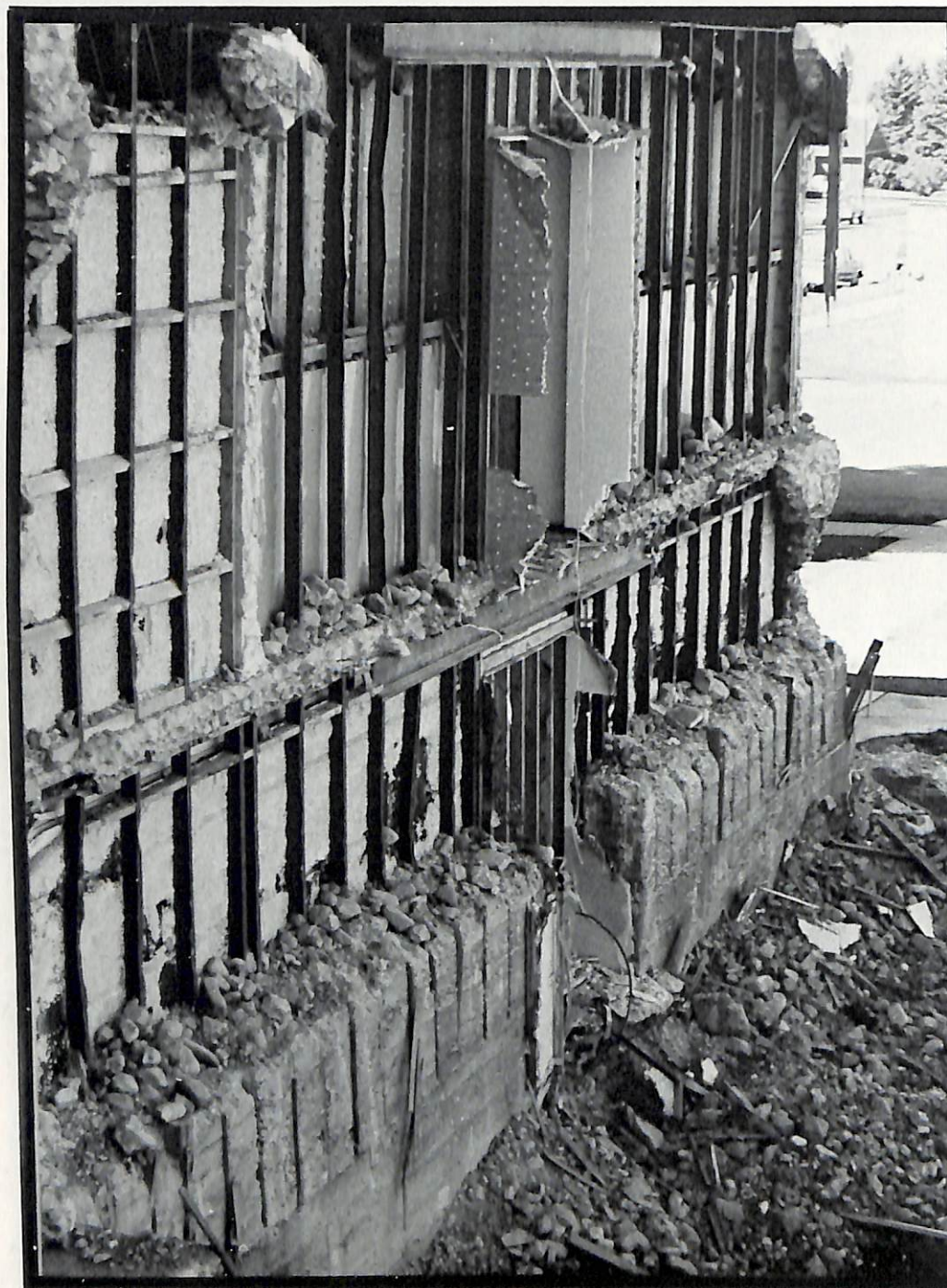
1. Demolition of the old rock building exposes concrete, stone, and metal framework. Drafts penetrate adjoining halls during the cold winter months. 2. This giant crane aids construction of the new shop building in Afton.
