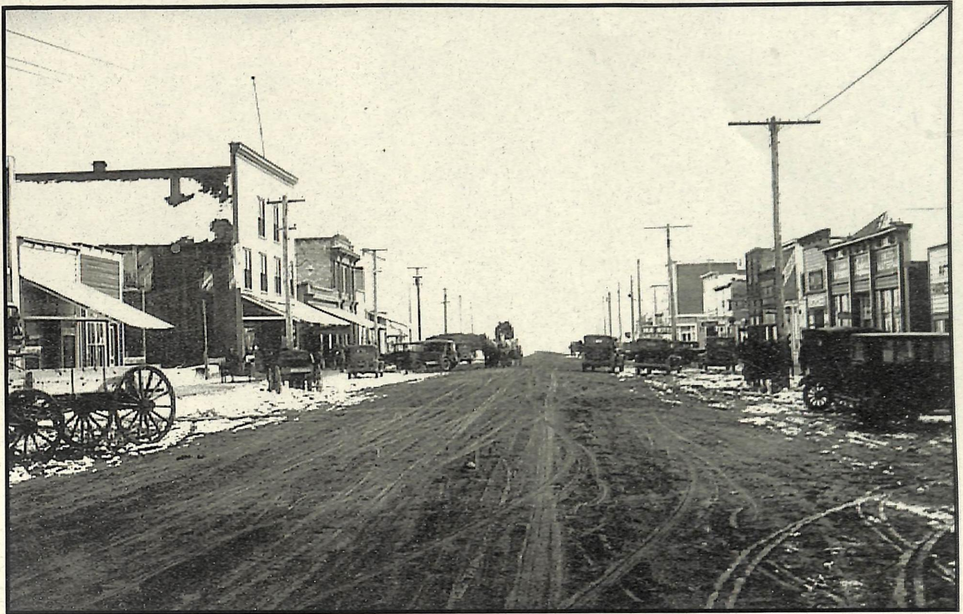
Afton Main Street Looking South
