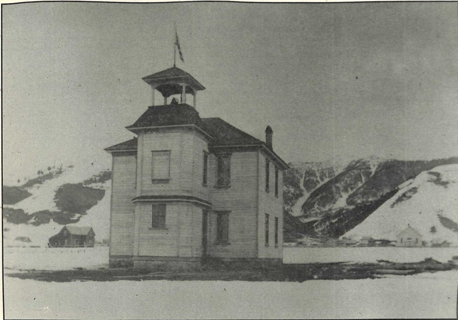
Grover School House built in 1900-1901. Gave 24 years of service.
