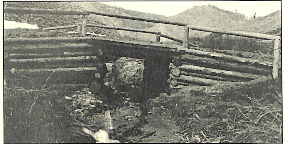
Bridge on the highway between Cokeville and Star Valley, 1917
