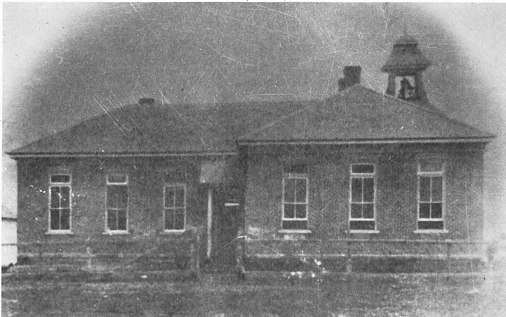
Fairview red brick school built in 1903 consisted of three rooms with a bell tower. The cost was $1,200. The bricks were made by William Brough, from Woodruff, Utah, at a kiln in Fairview. The school was in use for about 25 years.
