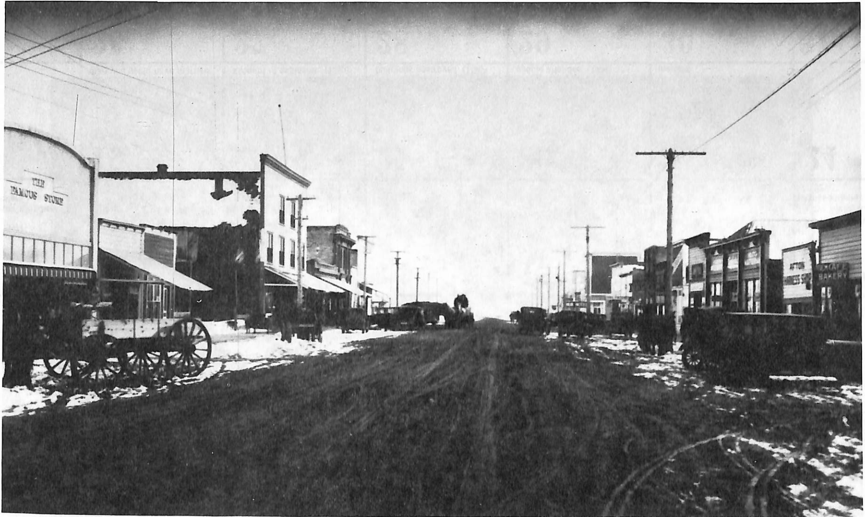
Looking South, Afton Main Street, date unknown.
