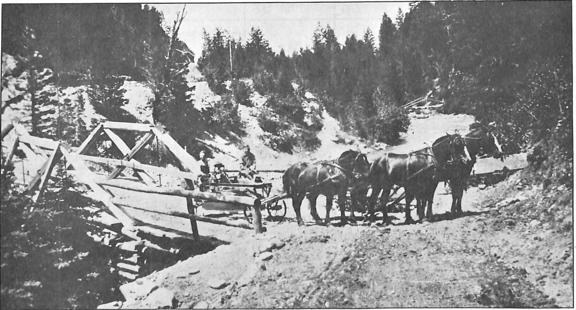
This is the beginning of the construction of the Greys River Road. The driver is Francis Simpson and Heb Merritt is on the grader. (1922-23)
