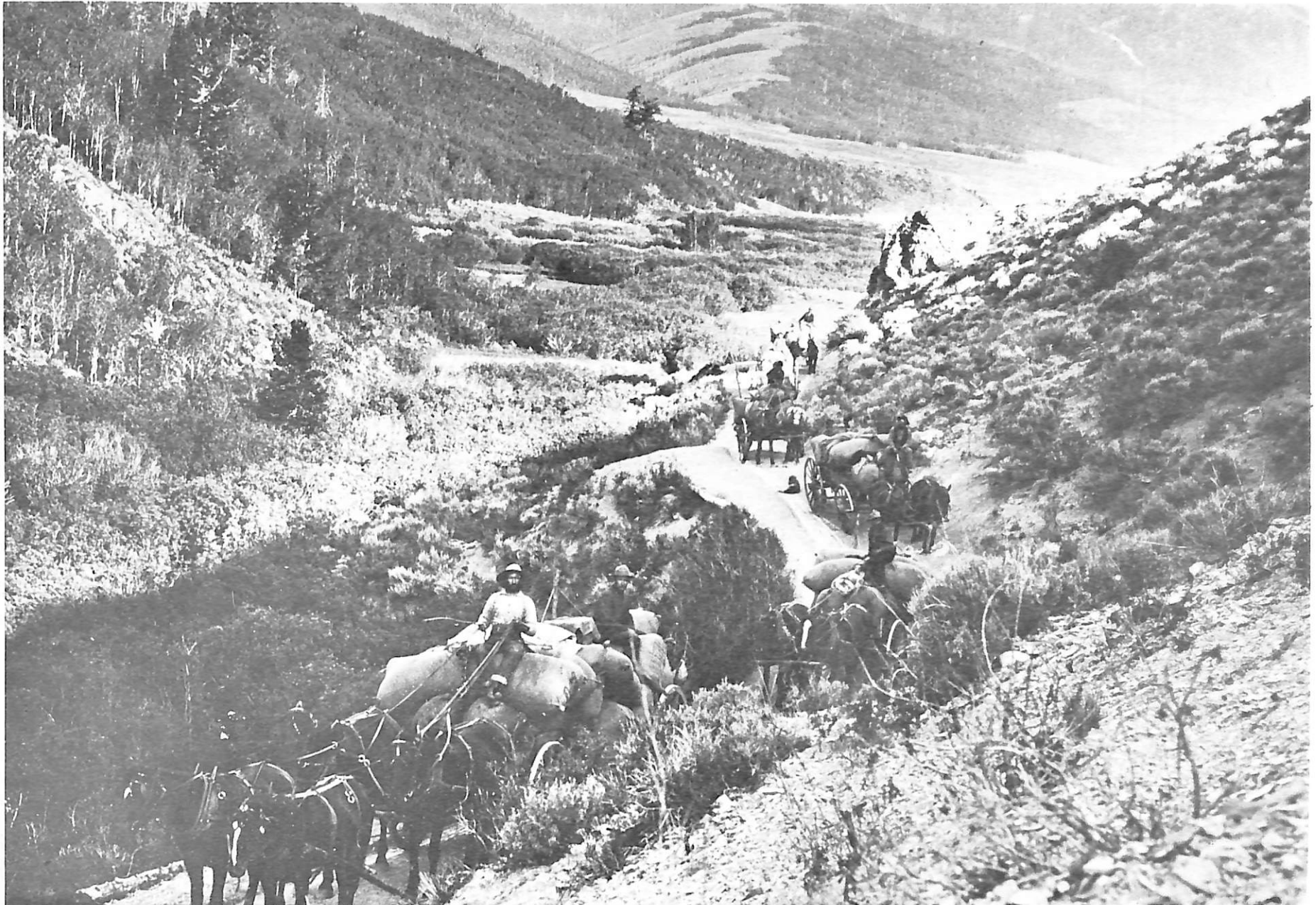
Freight train traveling the Crow Creek Road between Star Valley and Montpelier. Route was abandoned when the state of Idaho would not share in the upkeep of the road. The present South End Hiway was then constructed. The Star Valley Historical Society sponsored a trek to travel the road and visit the Halfway House during the summer of 1985. (Photo contributed by Ted Heiner.)
