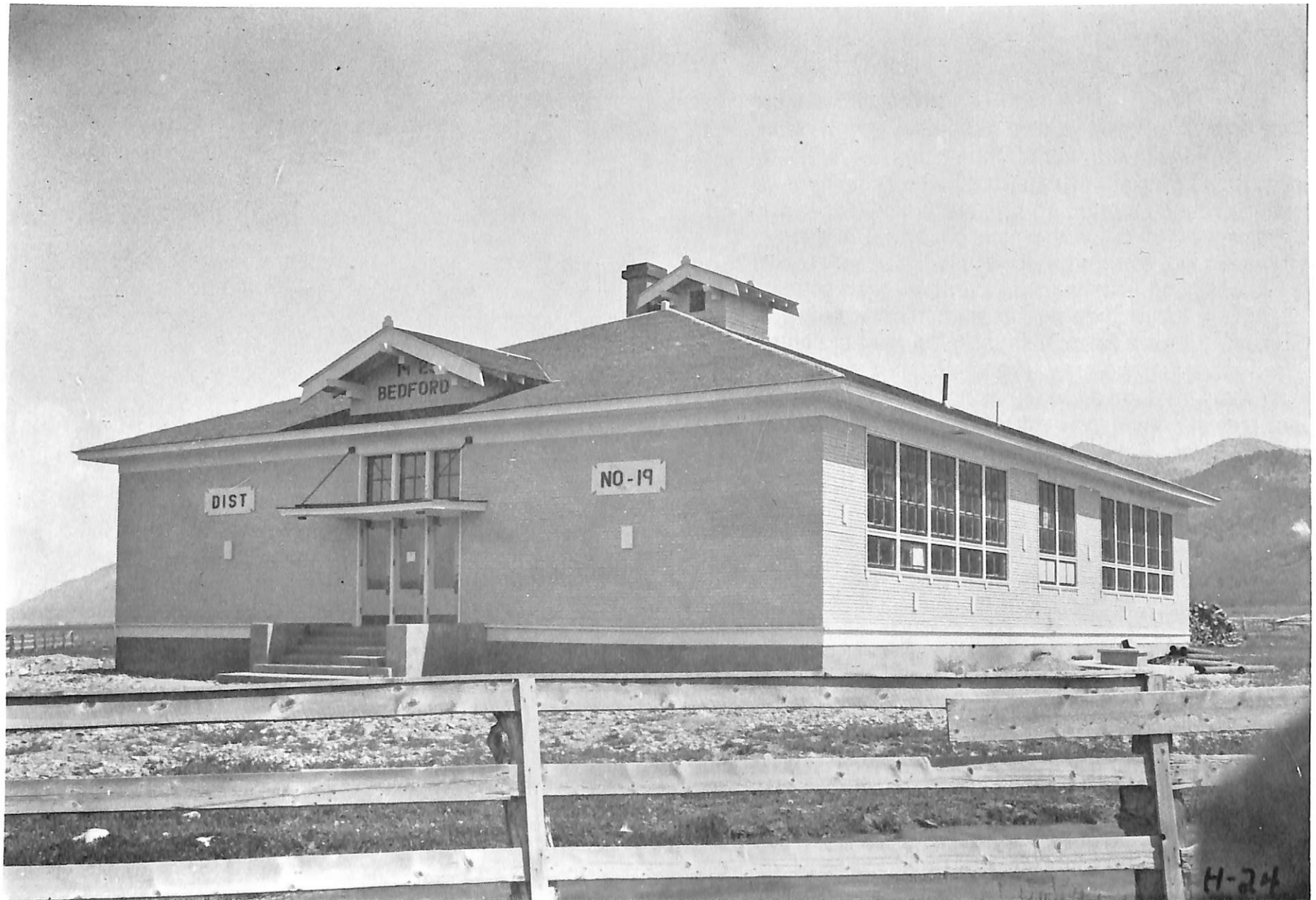
Newly constructed Bedford School, circa 1925
